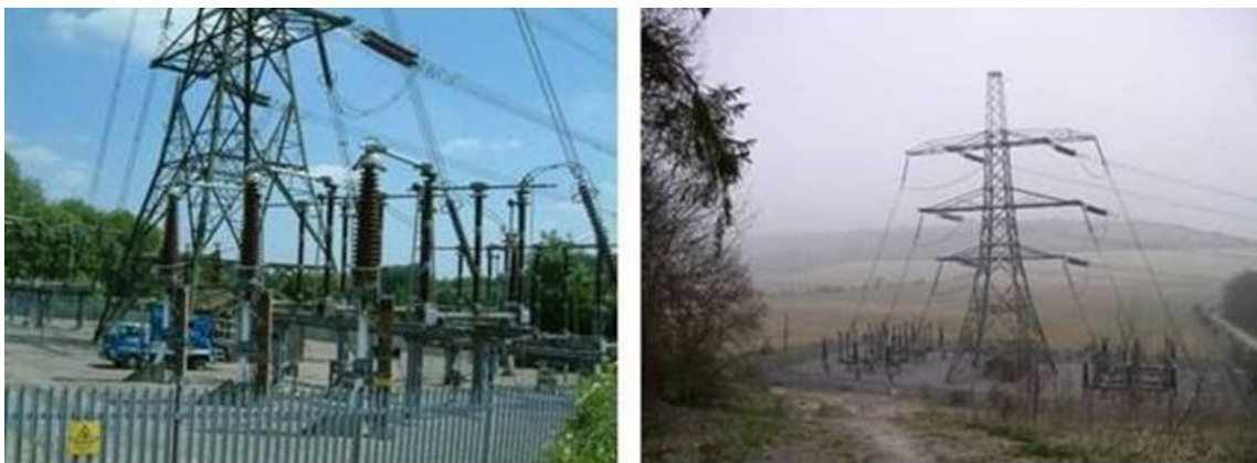
Figure C.5: Cable Sealing End Compounds
