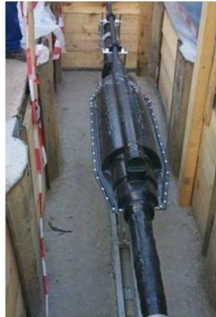
Figure C.2: Cable Cross-Section and Joint
